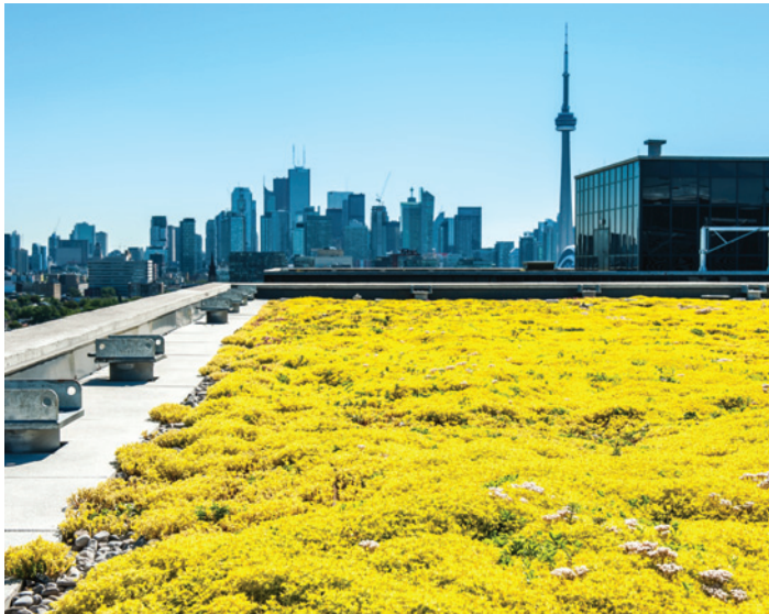
FIGURE 1 - A green roof installed on a high-rise building in Toronto. Photo courtesy of Greg Van Riel
