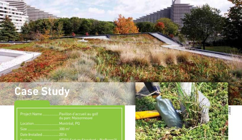
The Pavillon d'accueil au golf du parc Maisonneuve green roof features a "soilless" extensive system customized with the BioBerm™ option to create a meadow-like rooftop befitting the
